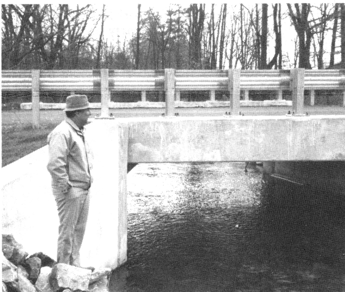
Rep. Semmel checks out bridge crossing Coplay Creek. The lawmaker was instrumental in helping to secure funding for the structure from the highway and bridge capitol budget.
