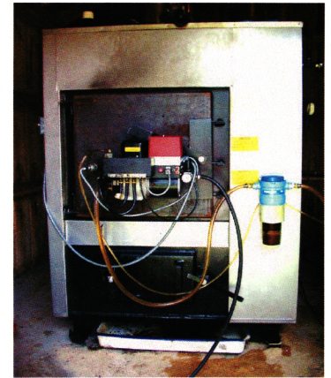
Above is a heater Brendle modified to run on vegetable oil
